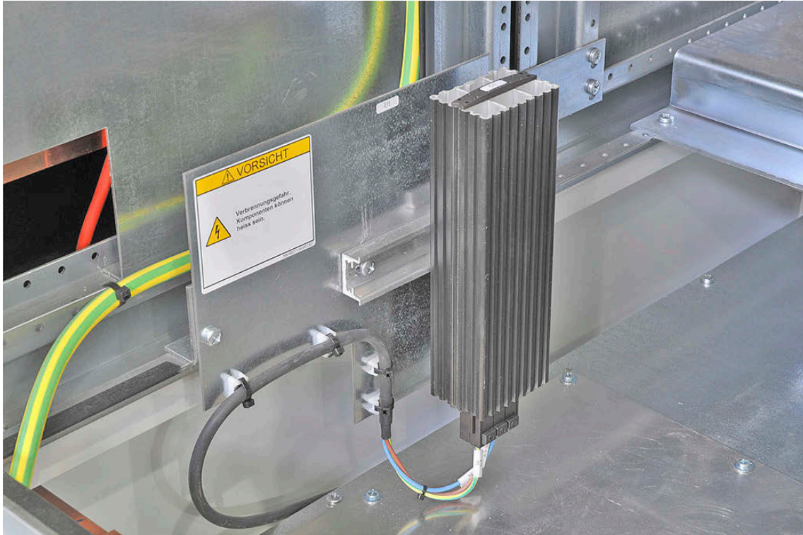
Figure 19 – Heating element
